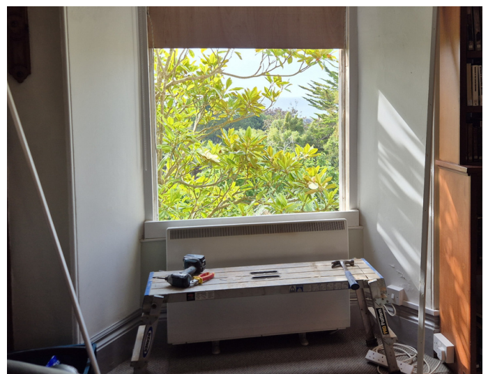
Window work in the Literature Room
